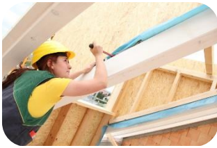
Picture 3: Lisa, carpenter (source: AMH)
